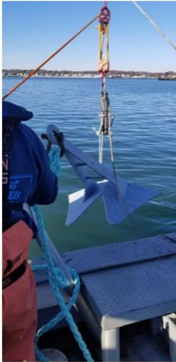
Photo 8: A 200-pound embedment anchor suspended and waiting to be deployed
