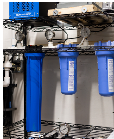
Left: UV filter Right: Filtration cartridges
