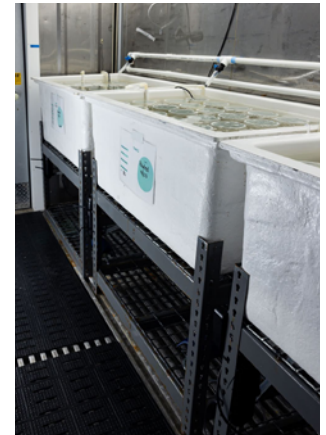
Left: Valve Right: Tank racks
